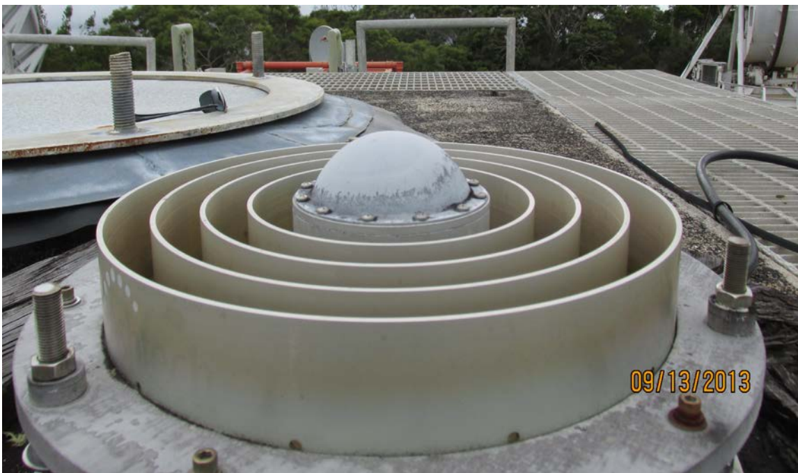
Figure 4 – IGS Tracking Station KOKB, view to the south.
