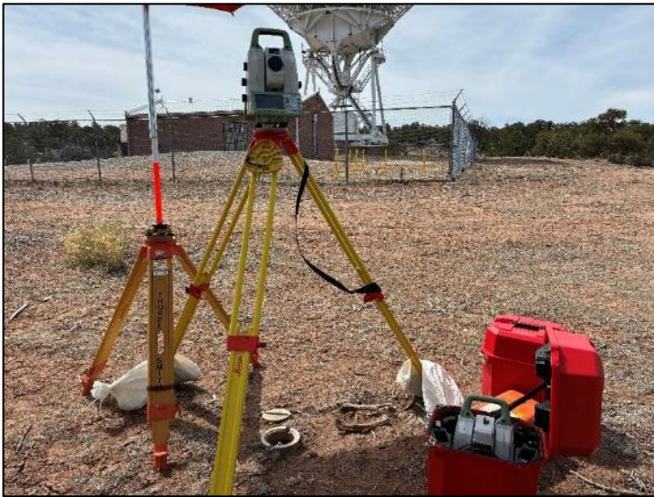
Surveying tripod for instrumentation
