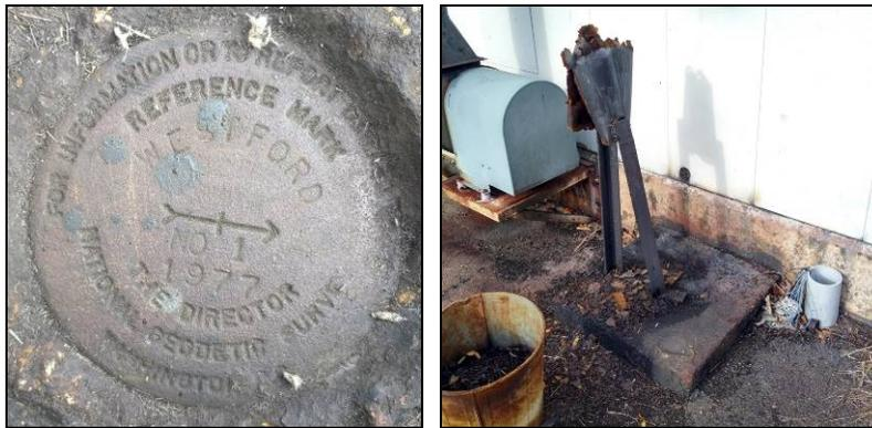
**WESTFORD RM2** is a National Geodetic Survey reference mark disk, stamped WESTFORD NO 2 1977, cemented in a drill hole in a 2 by 2 foot concrete pier that projects 3.3 feet above the ground surface. The datum point is a cross in the center of the disk.
