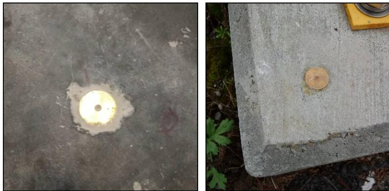
**NGS B** is a plug about 1.5 inch in diameter cemented in a drill hole in a concrete slab North of the VLBI radome enclosure and adjacent to the facility parking lot. No stamping.
