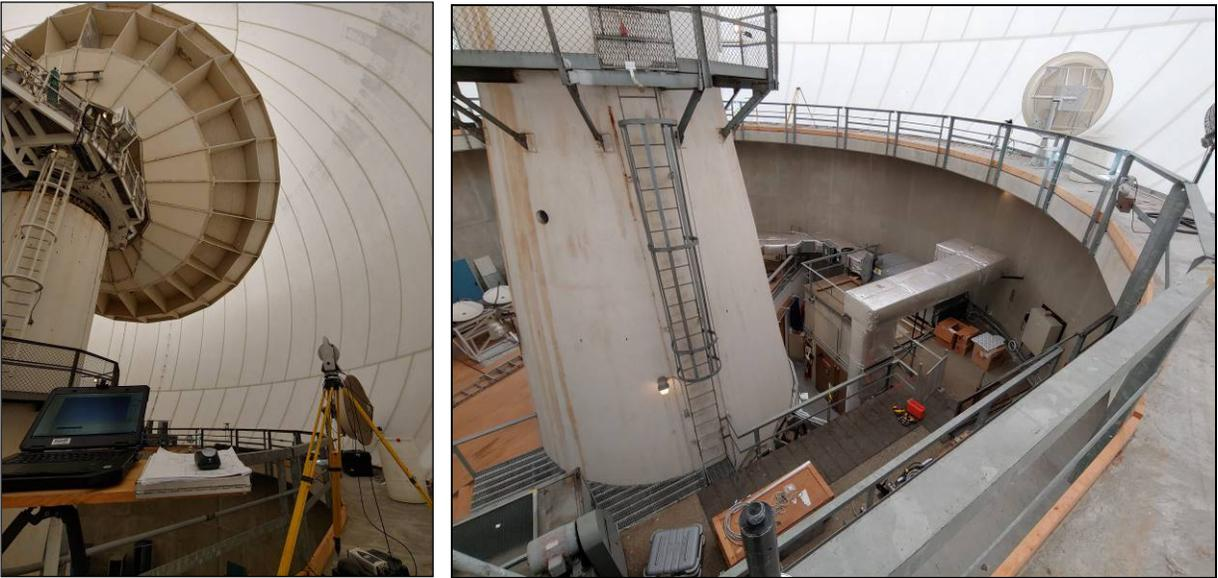
VLBI radio telescope 7209, mounted on a pedestal structure within a radome
