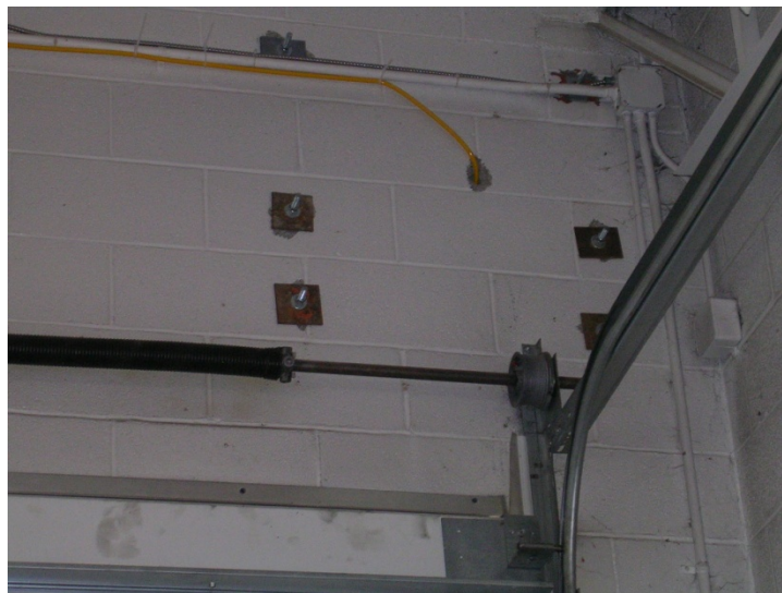
Figure 4 – Through-bolts with backing plates
