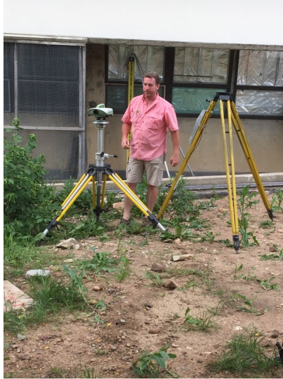
Figure 10. Leveling operations near Q407 (north side of Building 1). Q407 is visible on the wall just above the leveling unit.
