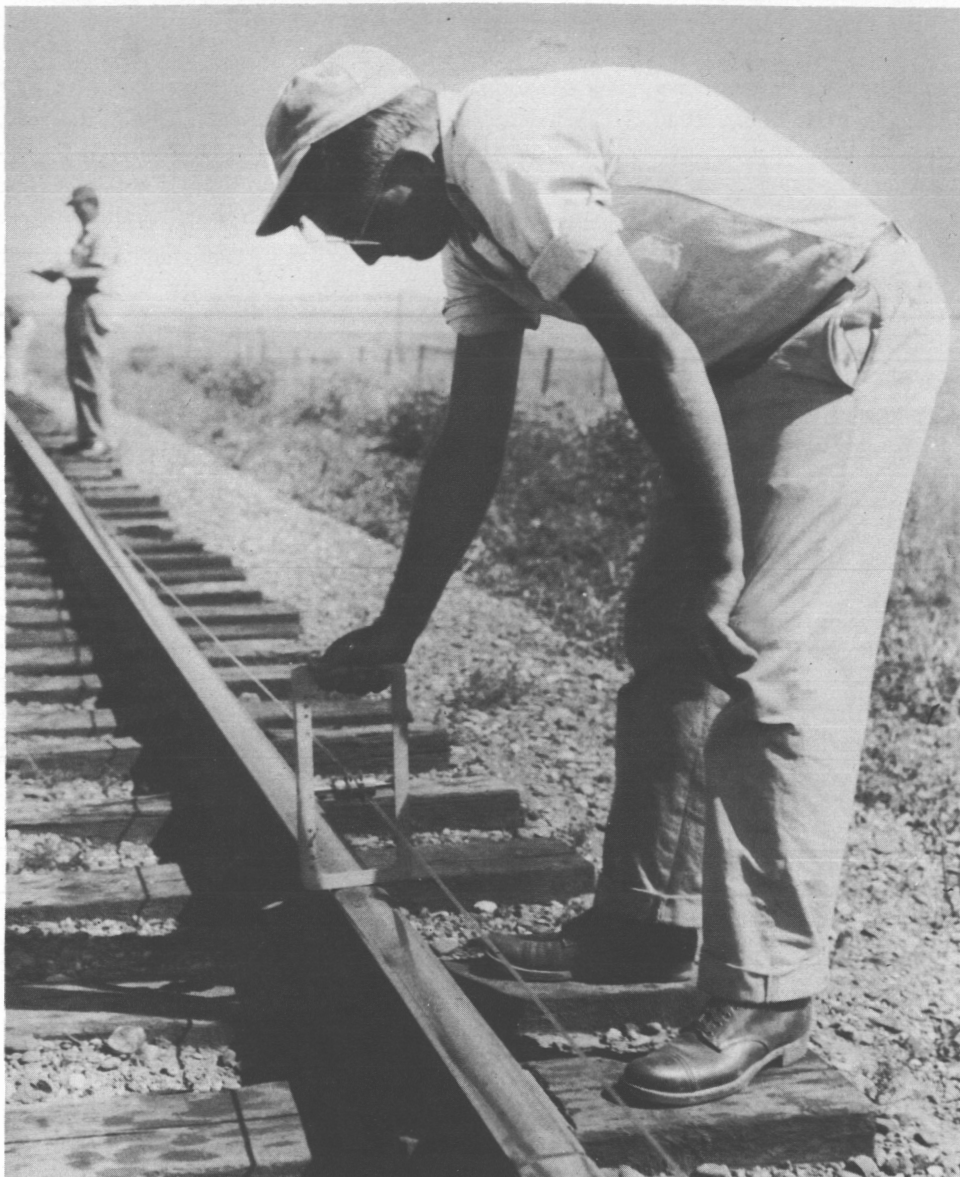
FIGURE 120.—Intermediate tape support, base measurement on rail.
