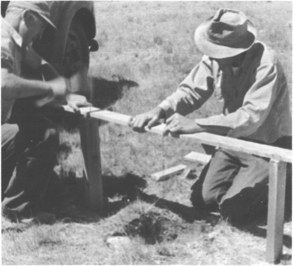
FIGURE 52.—Setting plumbing bench over underground mark.
