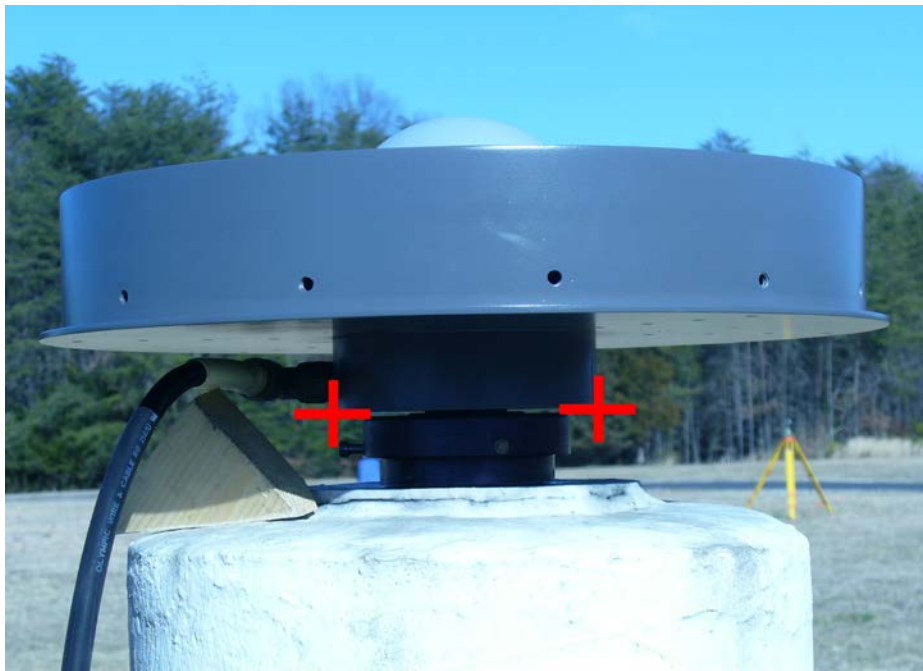
Figure 5 – “Zeroing out” the level instrument’s reticle on the mounting surface of the antenna (aka ARP) is achieved by raising or lowering the instrument; coarsely by adjusting the tripod height, and then a finely with the instrument’s footscrews. Independently leveling to both sides provides a clear target while eliminating any error due to any tilt or mis-level of the antenna.
